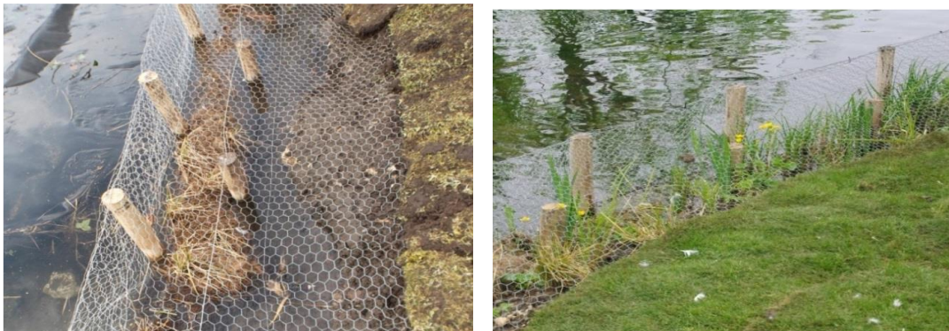
Example of bank restoration and marginal plants protected with netting (before and after establishment)
