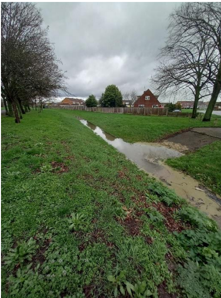
Water inlet at the west end of Canvey Lake, the Link Road entrance
