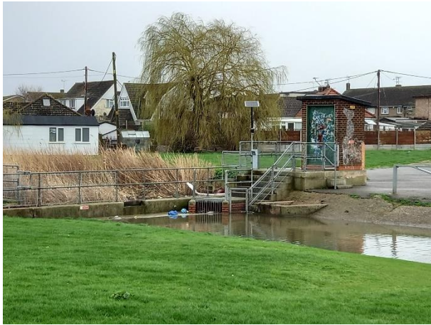
Environment Agency pumping station that moves water from the drains into the lake
